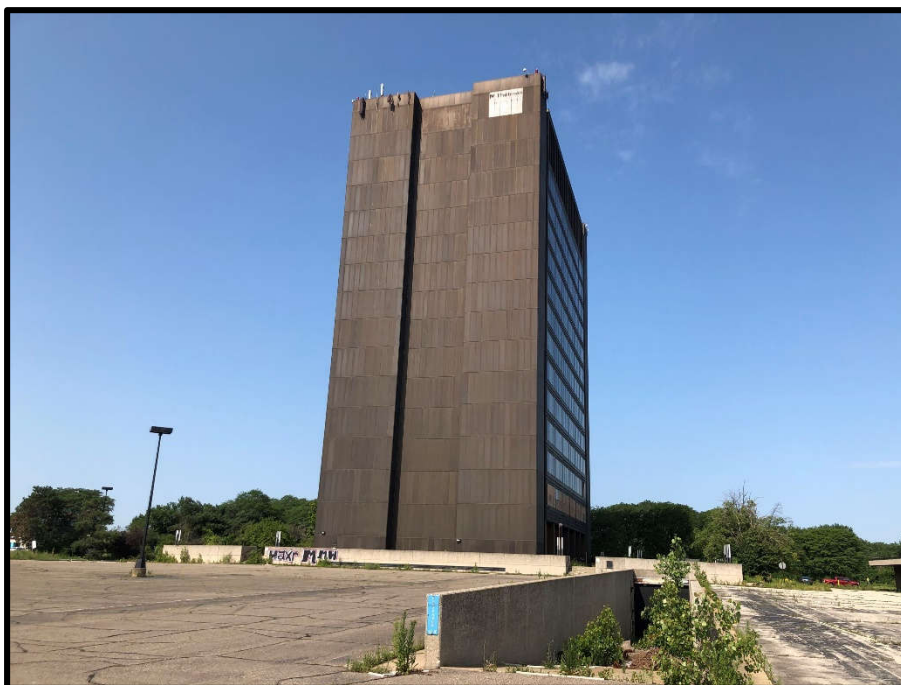
VIEW OF THE SUBJECT BUILDING FACING WEST
